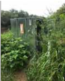
Overgrown vegetation needs trimming
