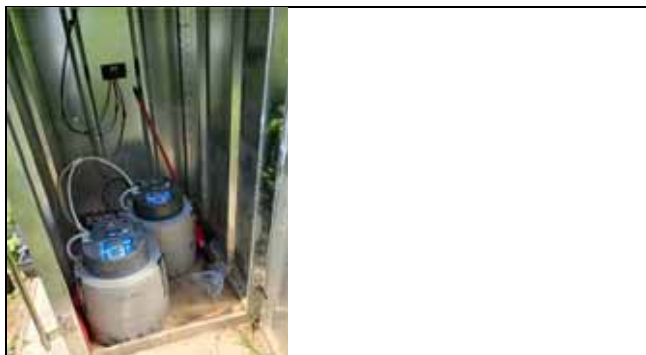
Inside of shed
